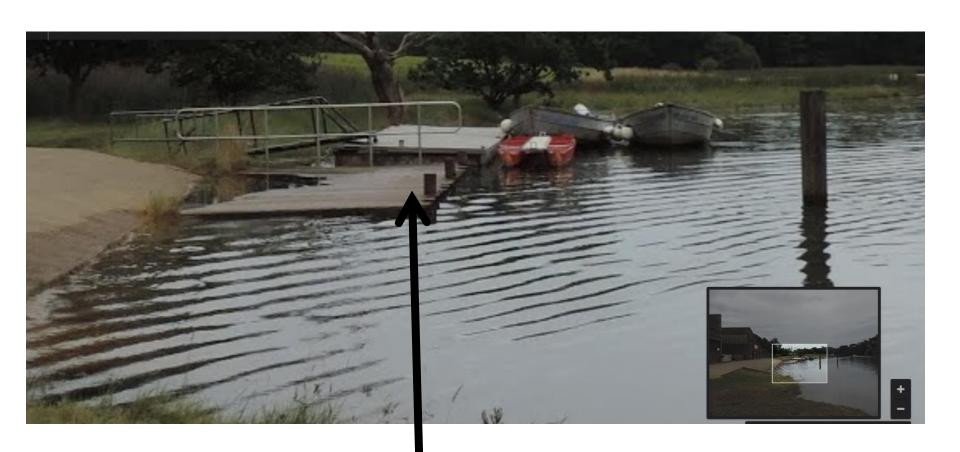
Pontoon will fix to this wall it has sheet pile on the waters edge fixings will be welded to this sheet pile
